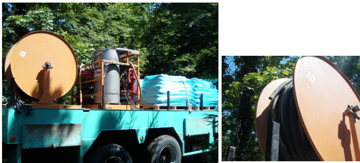
Figure 19 1 1/2" HDPE tremie pipe on a spool at the back of the truck. It is connected to the mixer near the supply of bagged silica sand and bentonite grout mix.
