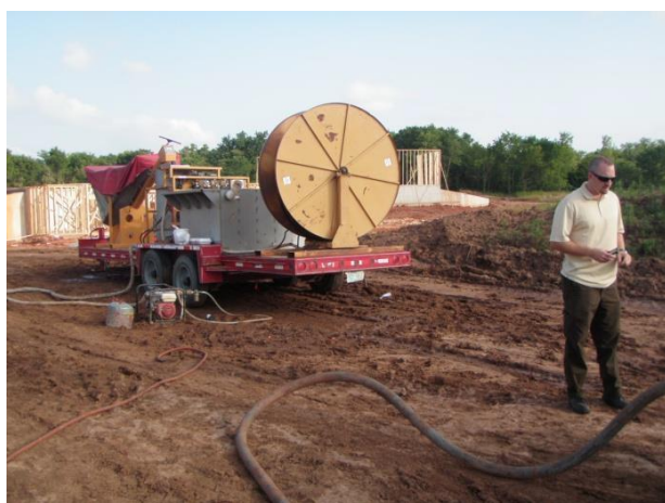
Figure 29 Left and Right: A grout rig "down south" in Oklahoma.
