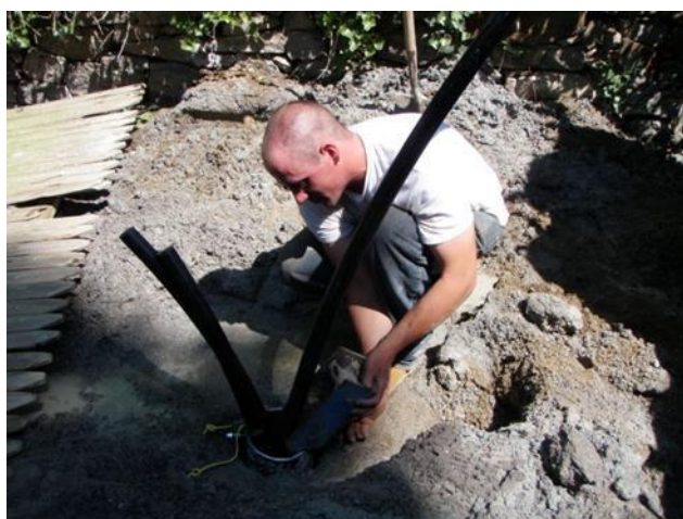
Figure 21 Twin rollers attached to the casing make insertion easier.
