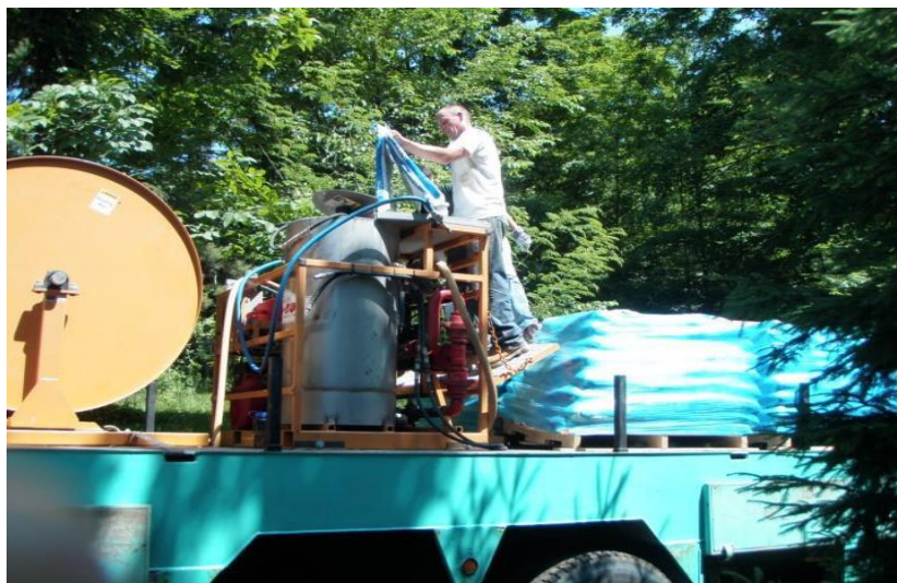
Figure 24 Adding silica sand and bentonite grout.
