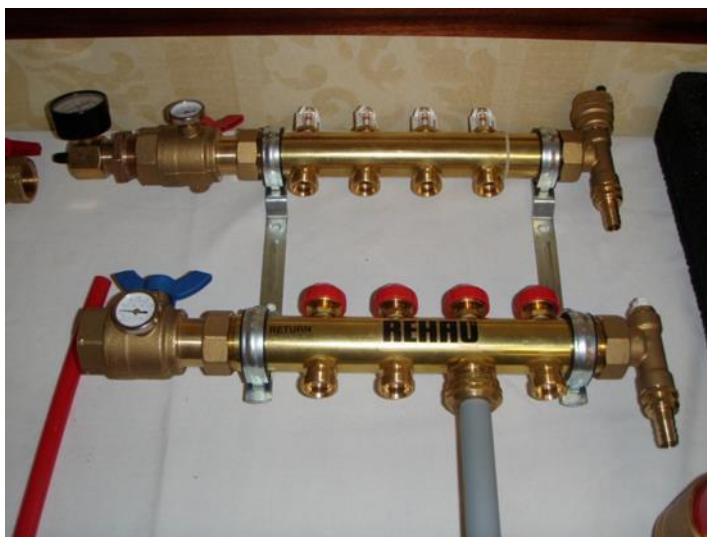
Figure 39 Prefabricated PEX pipe manifold.
