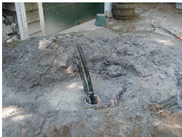
Figure 5 New England grey granite cuttings rise to the surface.
