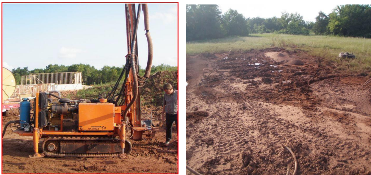
Figure 4 Boreholes in Oklahoma red clay by Track Drill, left, and the same filed with Loop Tails exposed, right.
