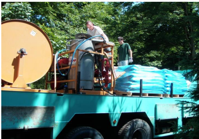
Figure 22 Grout is ready to be mixed and pumped in to borehole.
