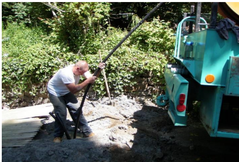
Figure 20 Tremie pipe pushed to the bottom of the 350' deep borehole.
