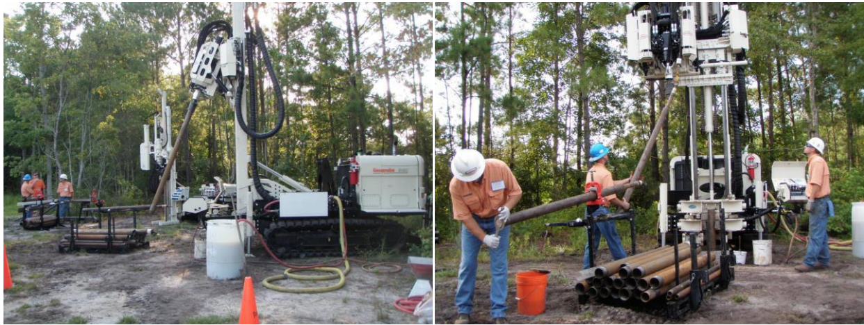
Figure 3 Demonstration of Coring Techniques with Percussion Drill, far left, and Sonic Drill, right.
