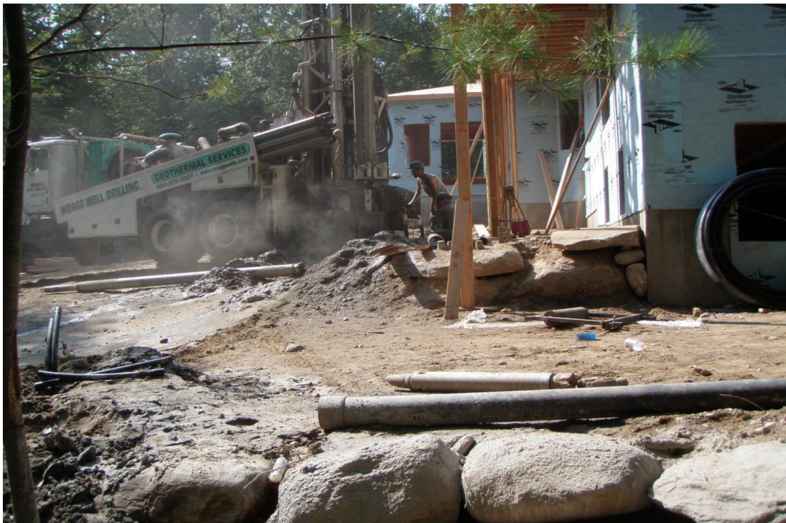
Figure 12 Typical drilling operation. This job was shown on the previous software sample (fig. 6) and site plan (fig. 7).
