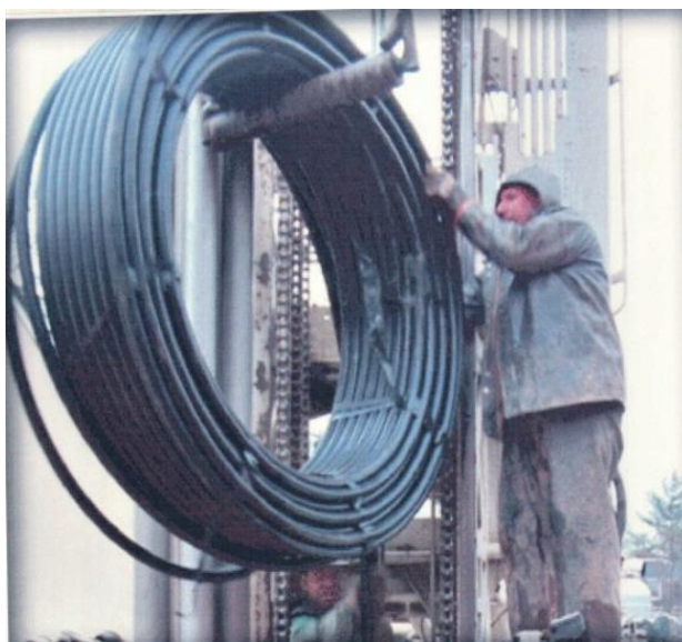
Figure 13 Driller uses roller sling for ease of operation.
