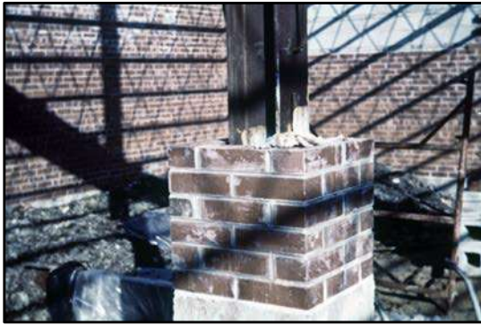
Photo No. 12 - Protecting a steel column from fire using masonry
