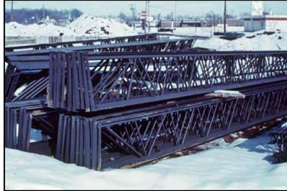
Photo No. 6 - Bar joists ready for delivery
