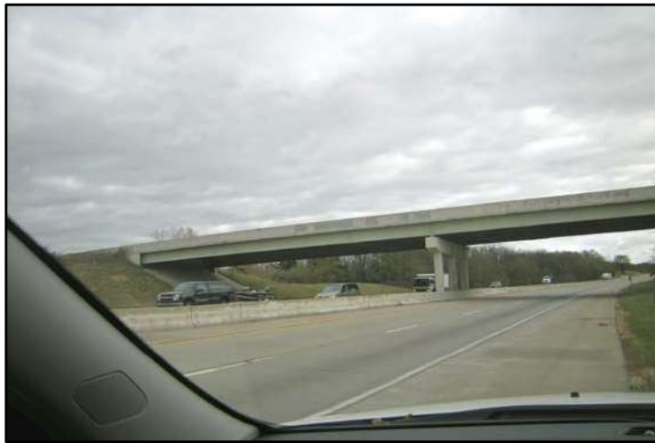
Photo No. 3 - Typical 2 span continuous bridge beam
