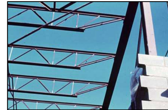
Photo No. 8 - Joists supported by a steel beam
