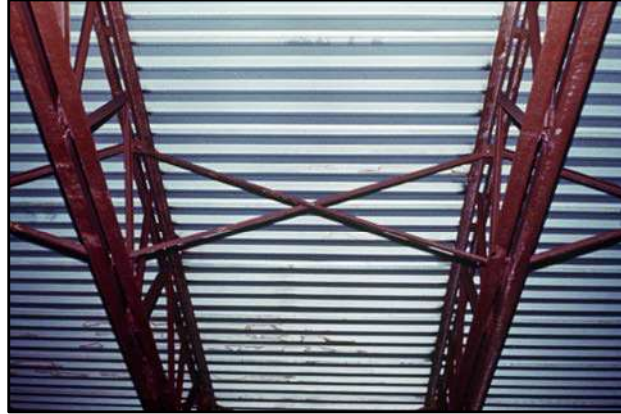
Photo No. 9 – Supporting metal decking
