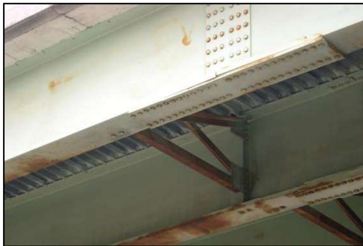
Photo No. 4 - Bolted connection on a steel bridge beam
