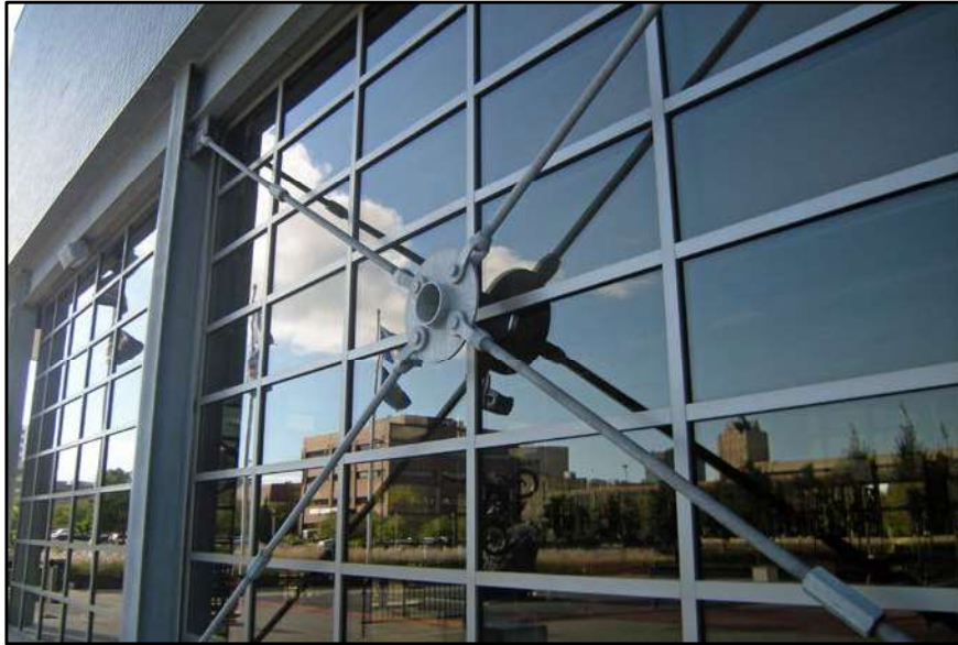
Photo No. 5 - Round bars bolted to center connection plate
