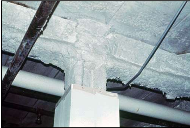
Photo No. 15 - Spray on fireproofing. Notice drywall protection for fireproofing which will be below the suspended ceiling
