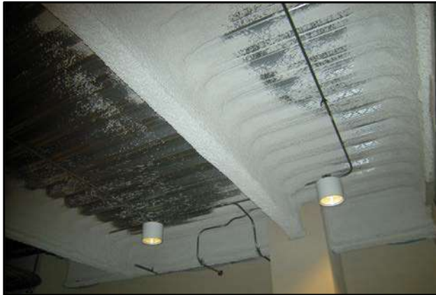
Photo No. 13 - Spray-on fire protection
