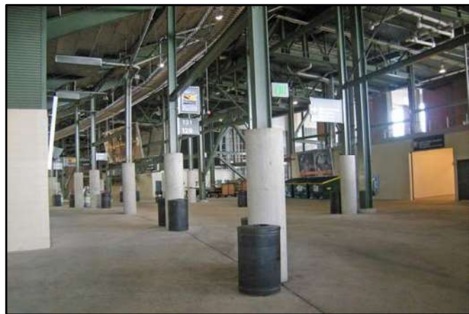
Photo No. 19 - Columns encased in concrete to protect them from physical damage
