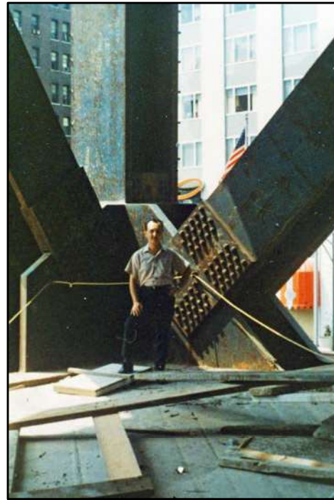
Photo No. 2 - Relative size of the welded corner joint for the John Hancock Building
