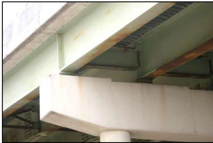
Photo No. 17 - Stiffener plate at support
