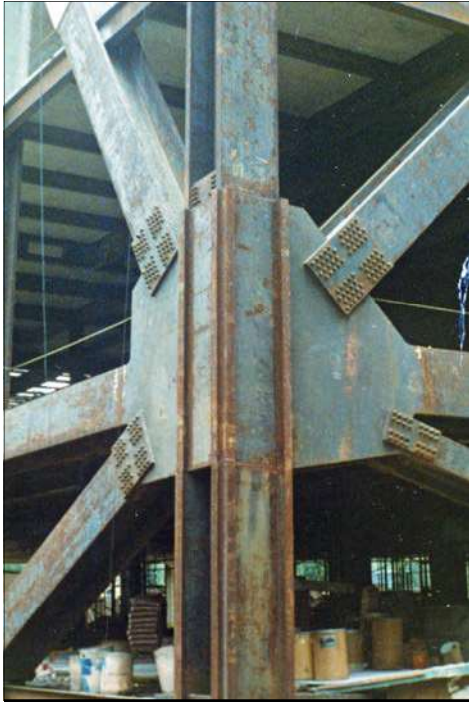
Photo No. 1 - Corner joint in John Hancock Building
