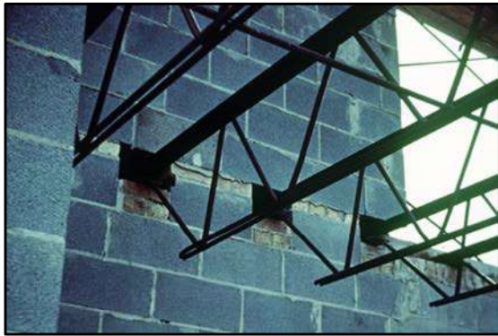
Photo No. 7 - Typical steel joists in masonry wall
