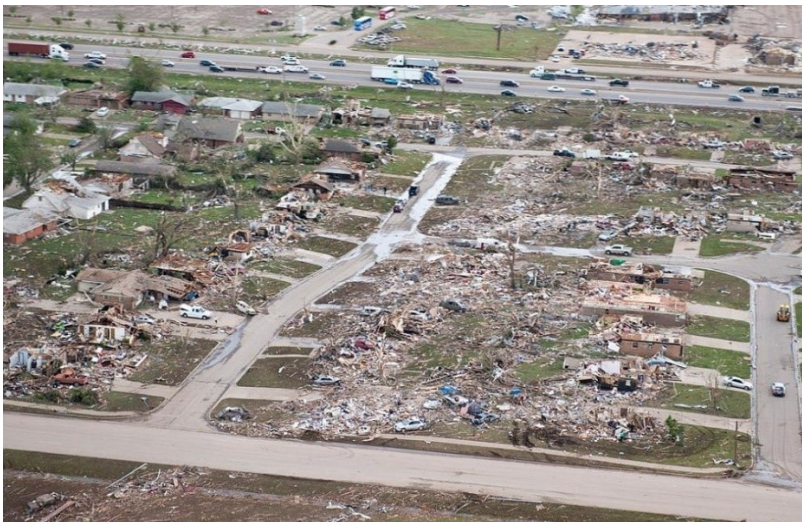
Flood and Tornado Damage aftermath (Wikimedia)
