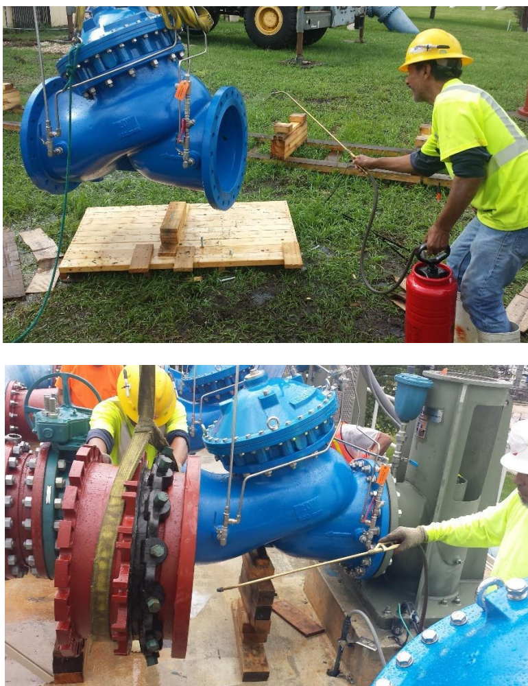
Figure 14: Examples of spray disinfection for pipe components being replaced on an existing finished water pump station. After being sprayed, the wetted surfaces should not be handled, and workers should wear rubber gloves.
