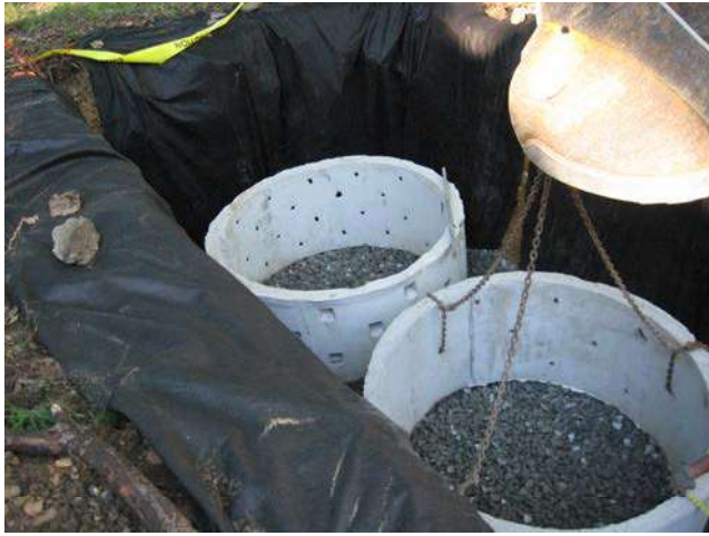
Recharge tanks placed within drywell.
