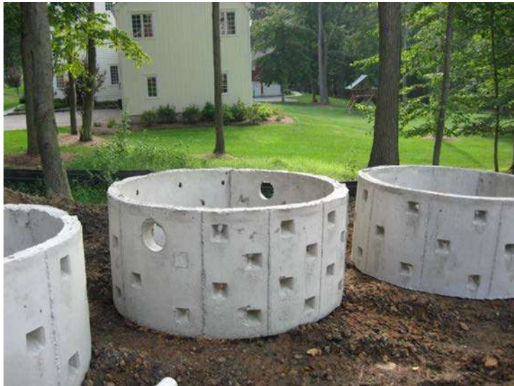
Recharge tanks awaiting placement.
