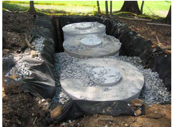
Recharge tanks installed with stone.
