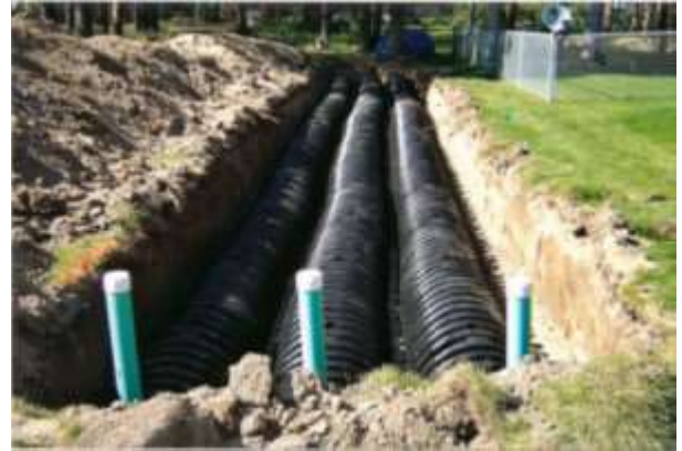
Infiltrator units placed in drywell.
