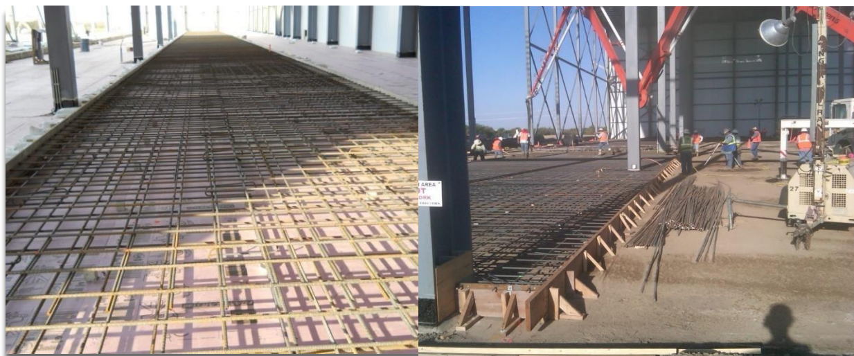
Figs. 45 & 46, Reinforces slabs that support racking that supports roof and braces walls (ACI 318 foundation design required). -15F freezer on left on insulation. 34F refrigerated space on right without insulation.
