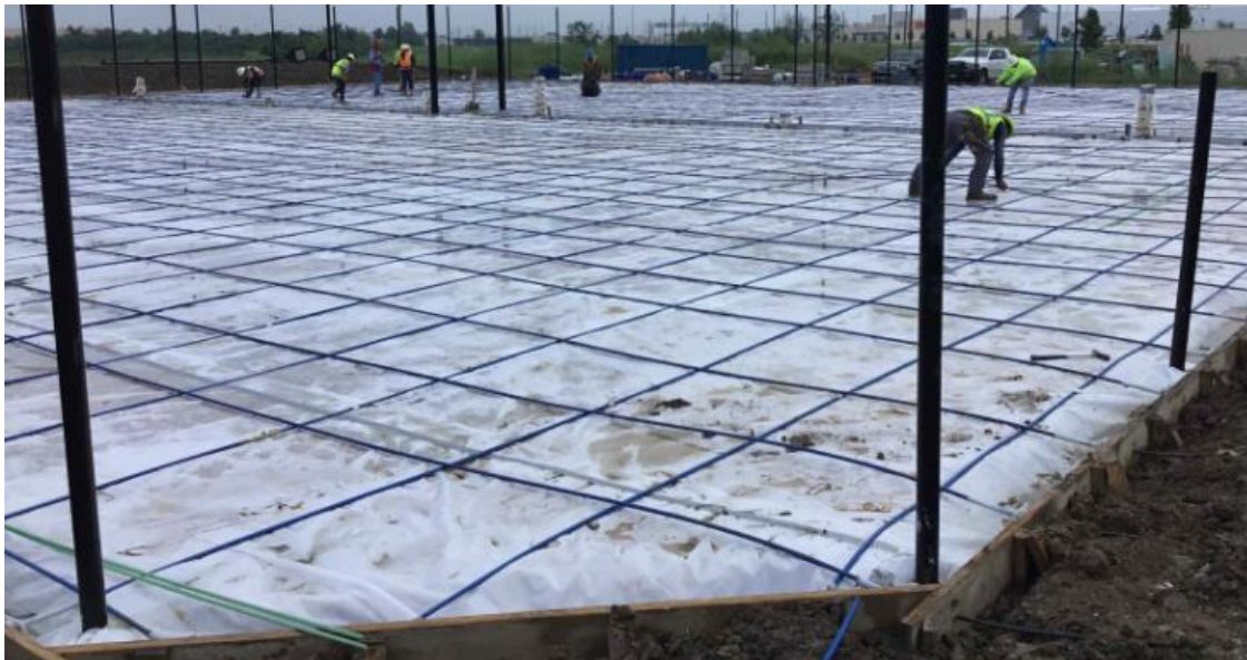
Fig. 23, Post-tensioning tendons in place over poly
