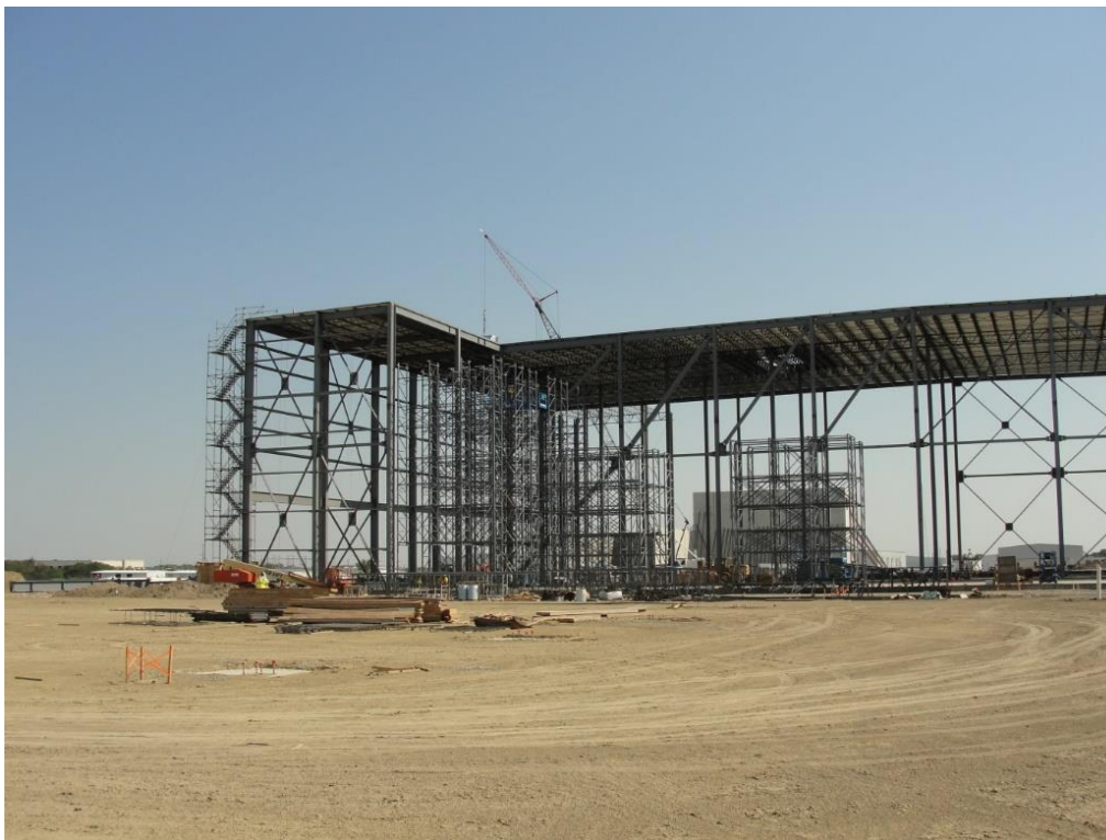
Fig. 39, Roof-supporting storage racking being placed adjacent to conventional steel-framed warehouse structure
