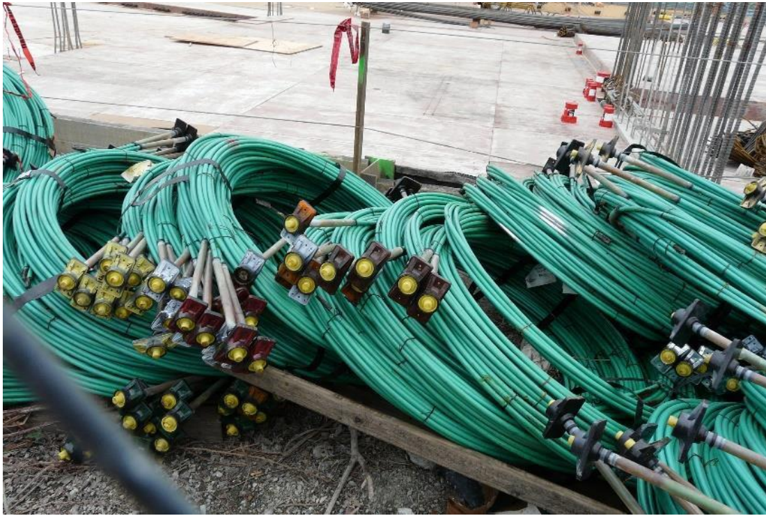
Fig. 22, Post-tensioning tendons ready to be placed
