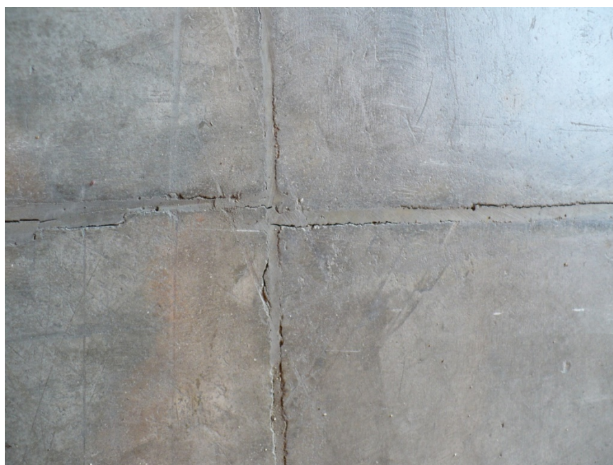
Fig. 50 - Joint filler in slab joints
