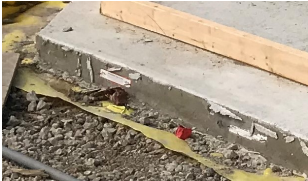
Fig. 37– Insert at edge of construction joint set into first concrete pour, with second concrete pour to follow. Square dowels shown to be placed at a construction joint placed in insert that was set into first concrete pour, with second concrete pour to follow ( https://www.pna-inc.com/products-designs/diamond-dowel-system )
