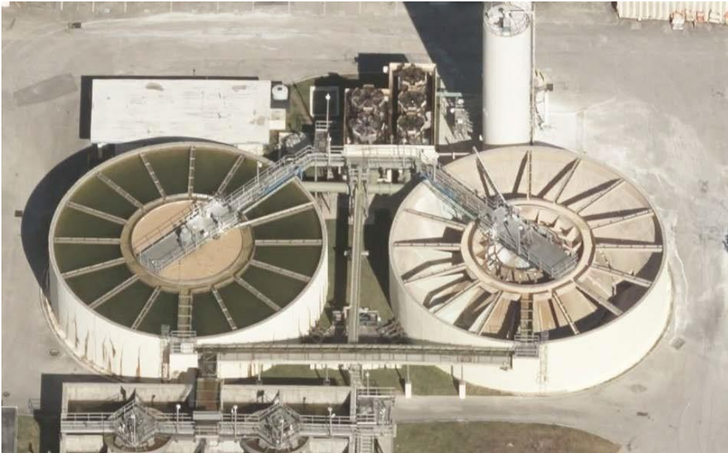
Figure 10: Example of two solids contact clarifiers for lime softening of water. Raw water is pumped into aerators (in the center) and then flows by gravity to the two clarifiers. Effluent flows by gravity to sand filters. The lime silos can be seen behind the empty clarifier.
