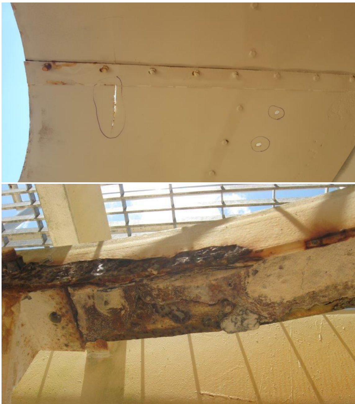
Figure 15: Solids contact clarifier with holes in the hood plates (top) and significant corrosion on the compression ring angles (bottom). These problems cannot be seen from the walkway, highlighting the need for an interior inspection.
