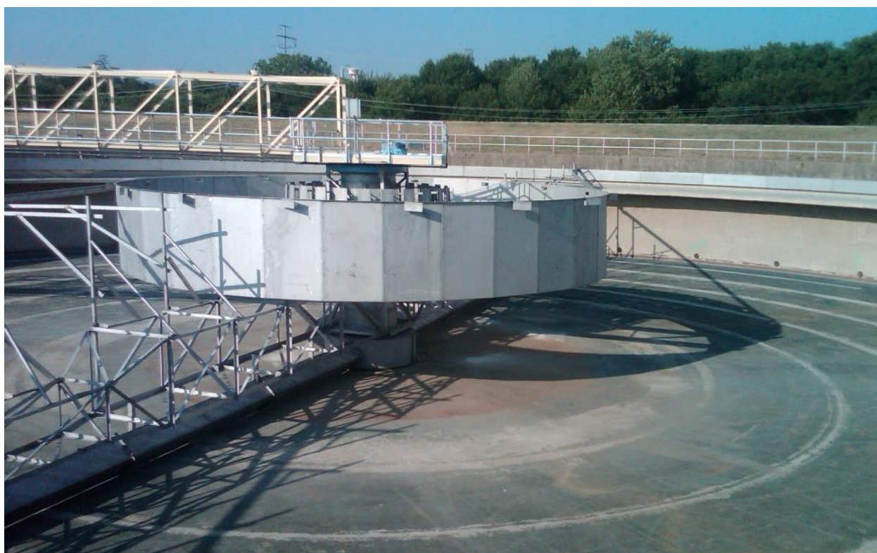
Figure 4: Internal components of a large circular secondary clarifier. In this case, all submerged components are stainless steel.
