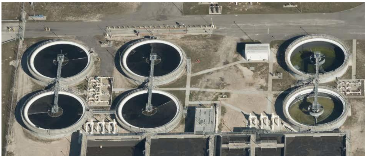
Figure 3: Six circular secondary clarifiers at a large WWTP. The large aeration basins (at the bottom of the image) discharge mixed liquor suspended solids (MLSS) to the six clarifiers by gravity.
