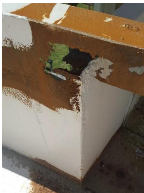
Figure 32: Example of thin steel discovered during construction after sandblasting.
