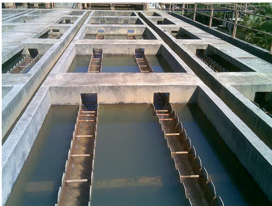
Figure 7: Rectangular clarifiers with effluent troughs.
