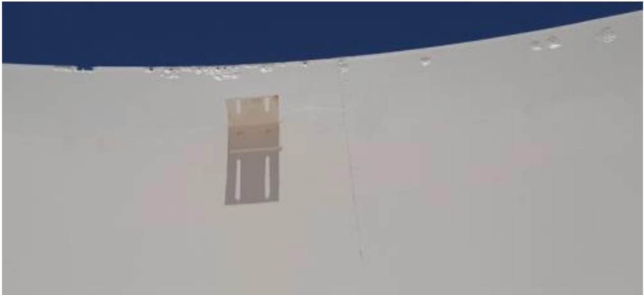
Figure 18: Depressions and holes near the top of the tank wall.
