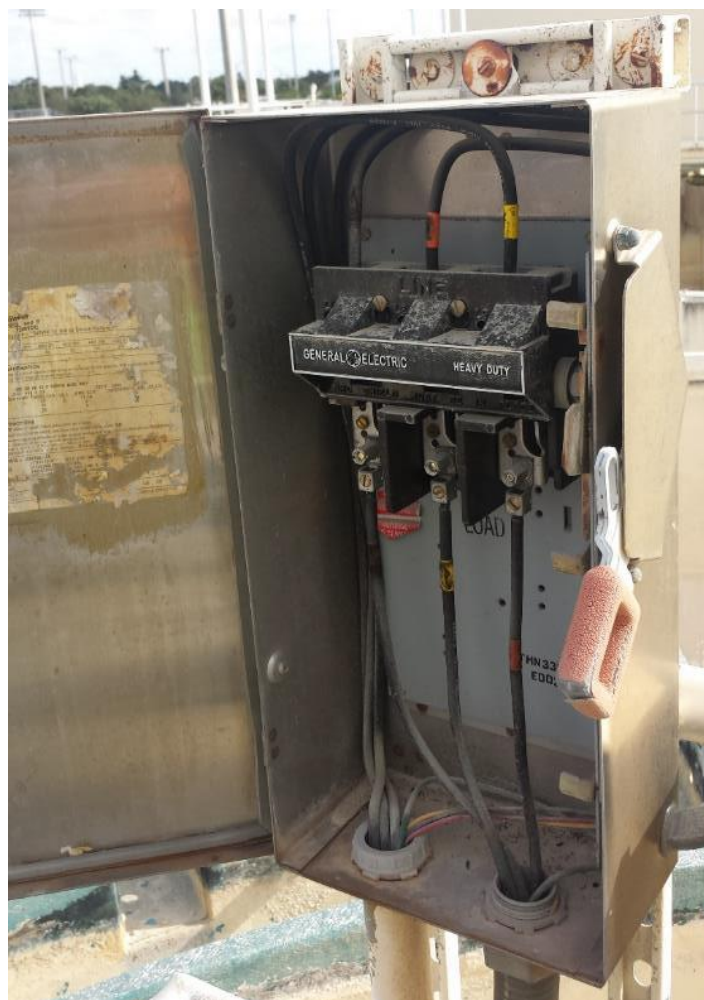
Figure 25: A 30-year-old disconnect switch on a clarifier.
