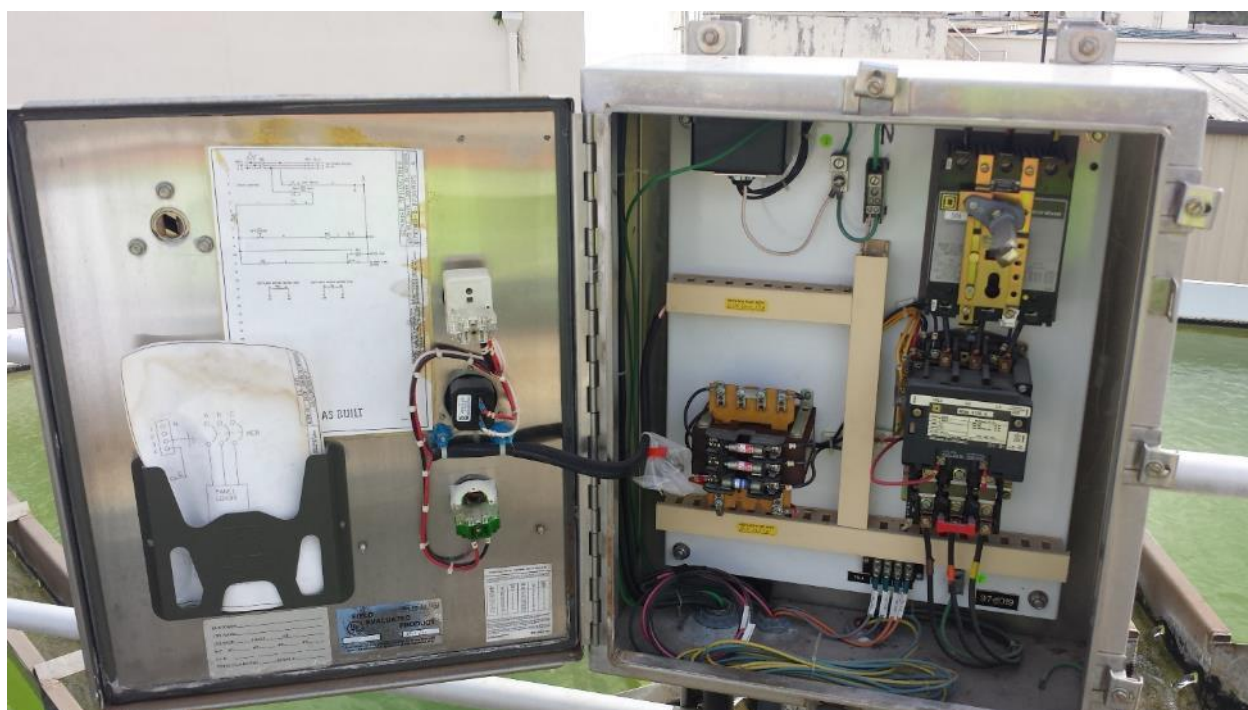
Figure 24: A 15-year-old control panel on a clarifier.
