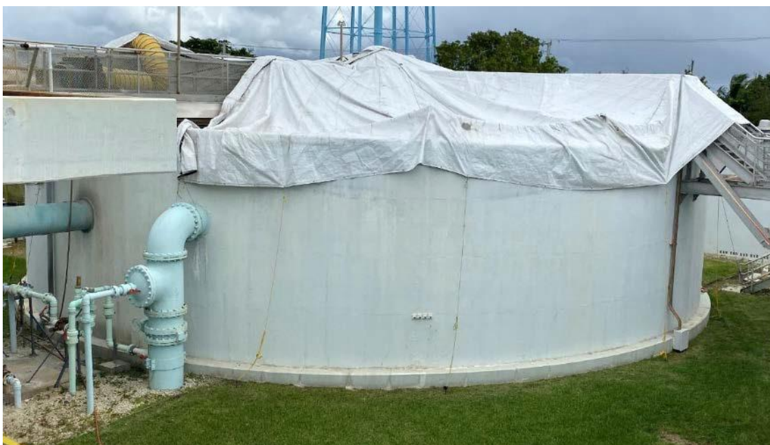
Figure 35: Example of a tarp cover on a clarifier. The cover functions to provide ideal conditions for blasting and coating carbon steel surfaces and provides dust control.
