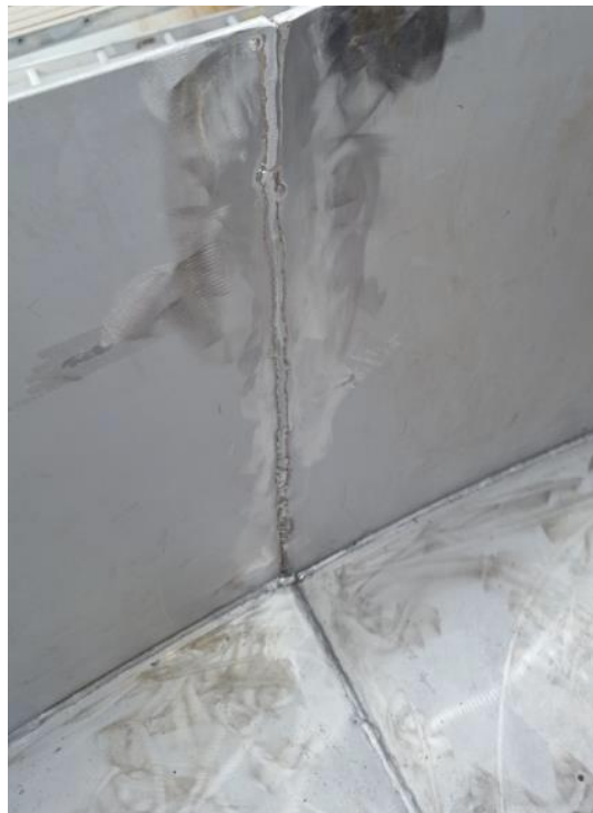
Figure 45: Stainless steel welds after grinding, smoothing, and passivating.
