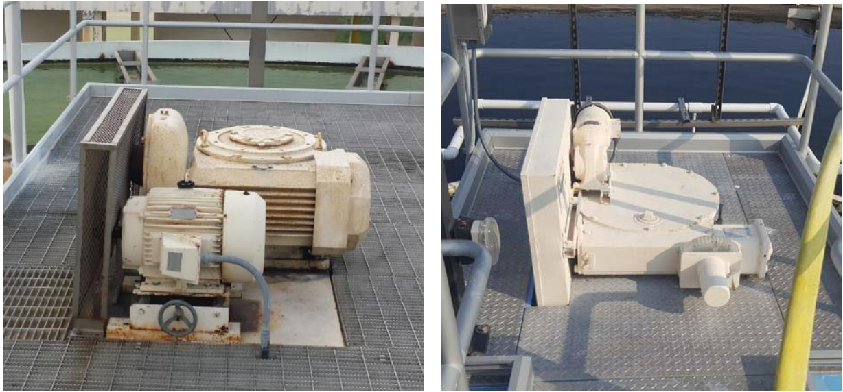
Figure 12: Compression ring supported drive for a solids contact clarifier (left) and a bridge supported drive for a secondary clarifier (right).
