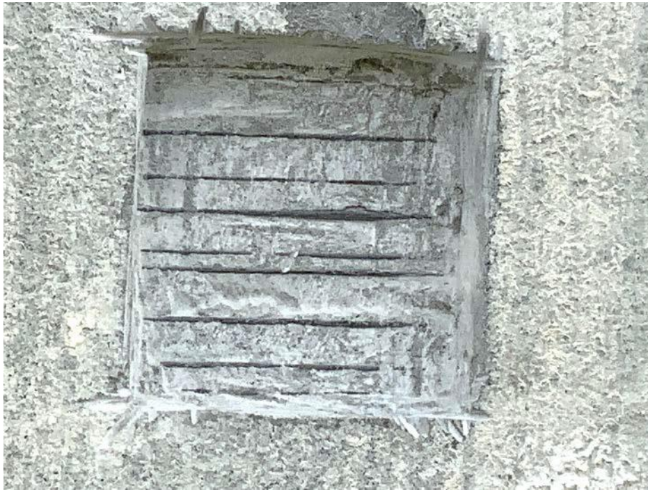
Figure 23: Surface removal panel on the outside wall of a 40-year-old prestressed concrete tank. The wires are observed to be in good condition.
