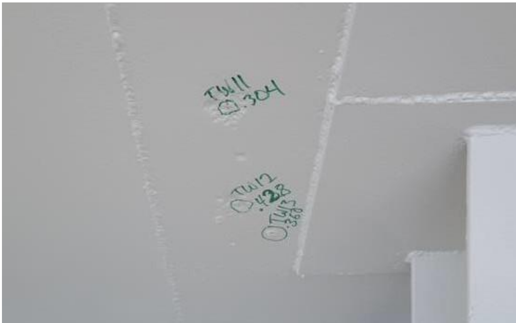
Figure 19: Bottom of a tank wall with the three depressions circled and steel thickness measurements written in green.
