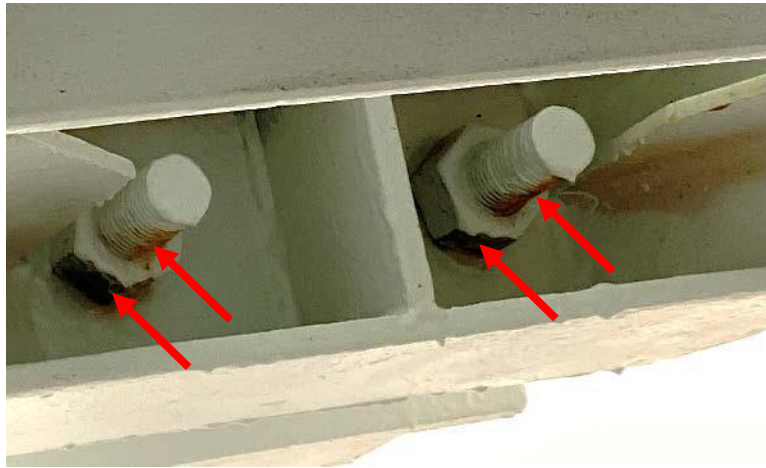
Figure 41: The red arrows point to steel surfaces without proper coating.
