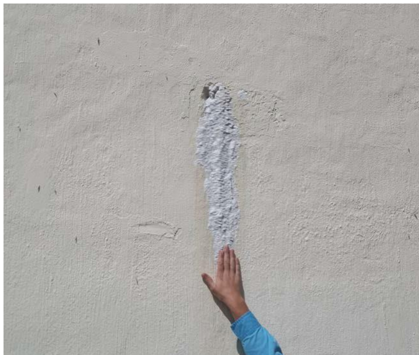
Figure 21: Example of efflorescence on the outside of a tank wall.
