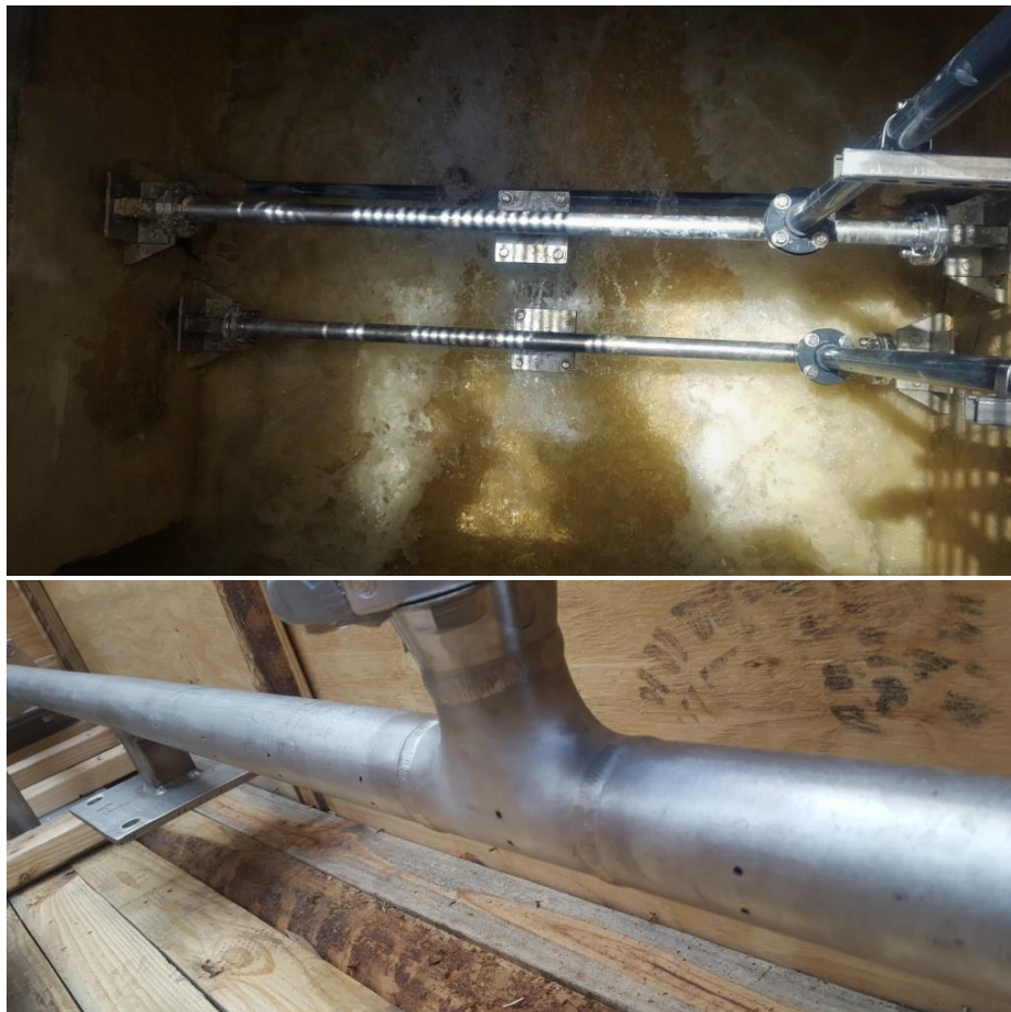
Figure 21: Examples of open channel diffusers.
