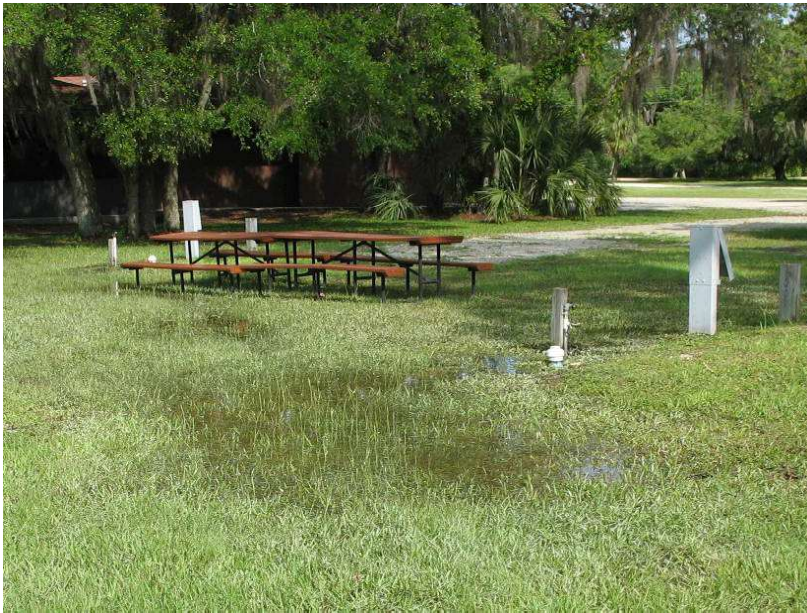
Poor drainage at campsite - notice utility services are located in standing water
