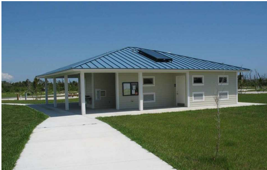
Bathhouse with solar water heater placed on roof. Also notice the information board on the wall
