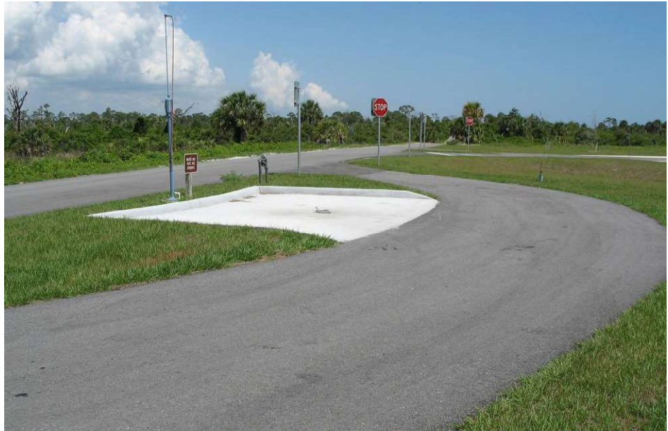
Examples of dump stations found in various campgrounds
