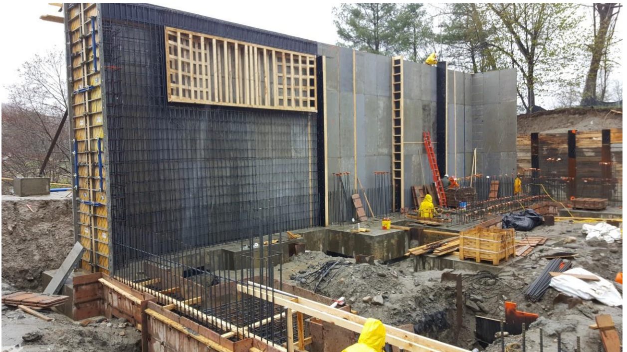
Large Louver Opening in a Wall
