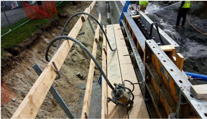
Vibrating Tool ready for use. Might not be inspected by rebar inspector.
