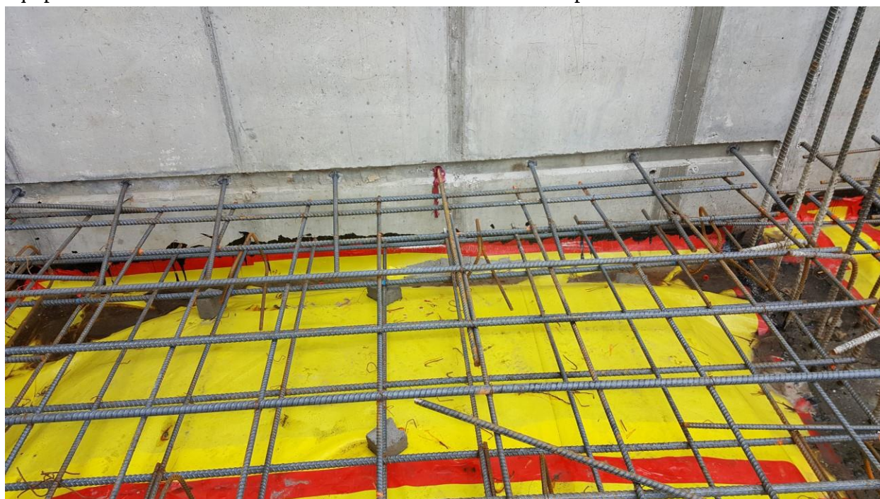
14" thick slab on grade with top and bottom Rebar mats and wall dowels
