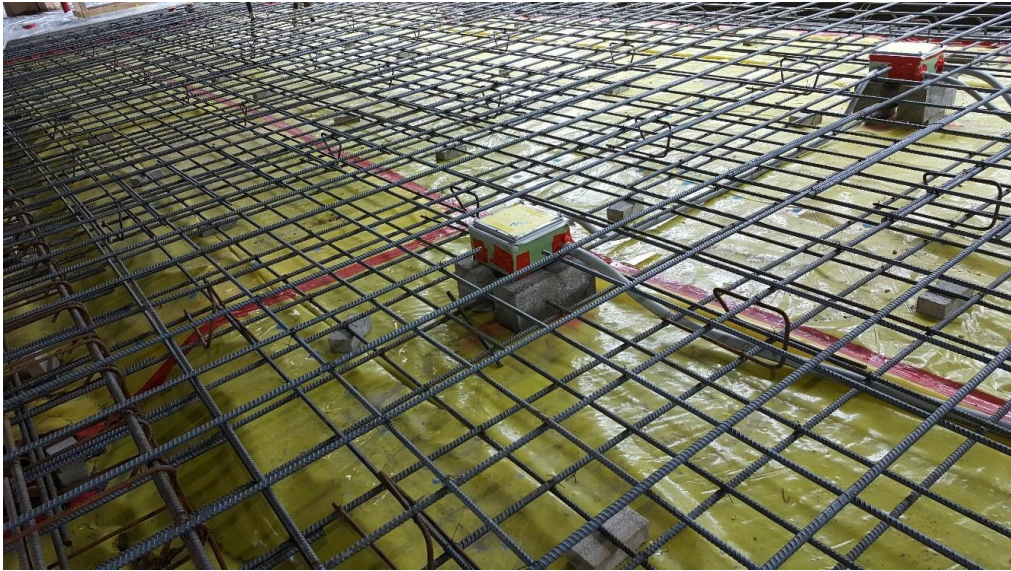
Slab with grade beams in lower left and upper right. #6 at 12" in direction of span. Utility boxes are mounted on big 4000 psi blocks. Rebar on 4000 psi bricks.
