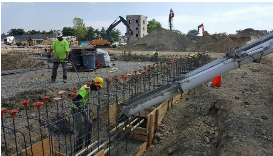
Vibrator used on a different job (after rebar approval)
