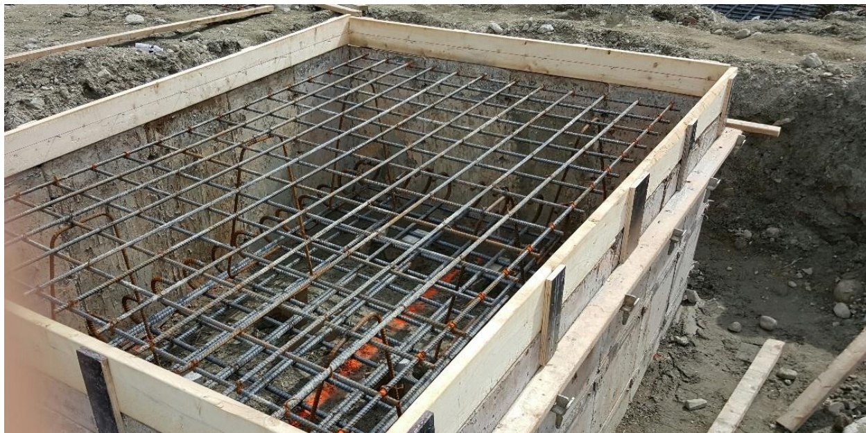
Top and Bottom Grid of Rebars in both directions- ready for concrete
