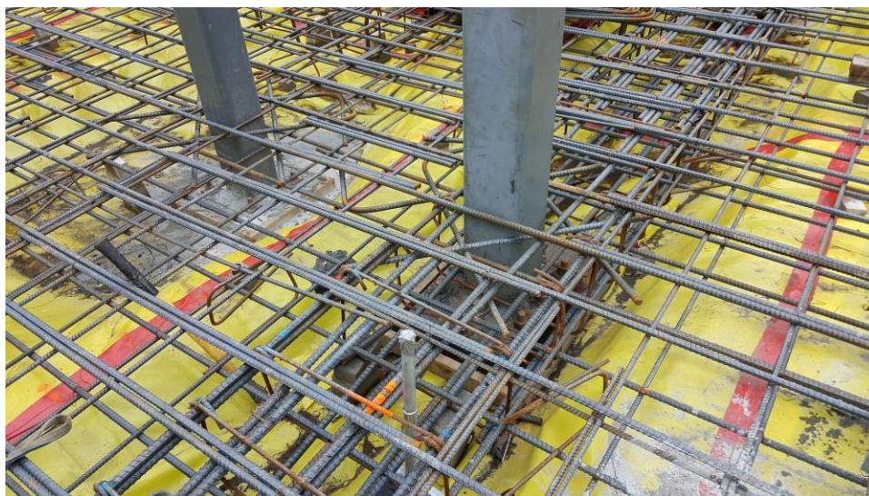
Grade Beam rebar across steel column base in slab on grade
