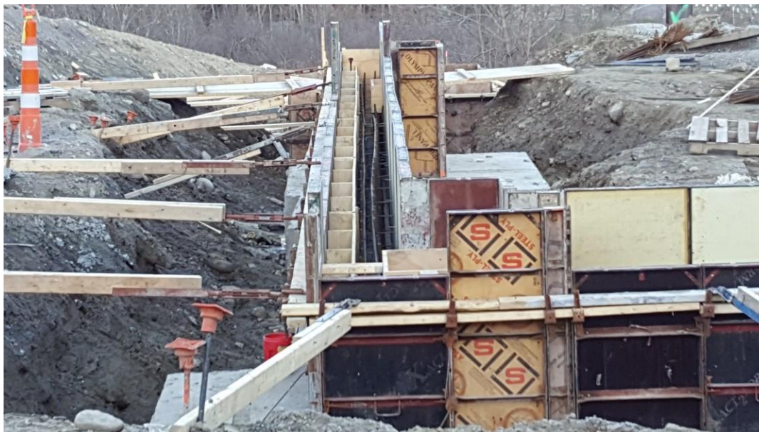
Short Wall inspected from above.
