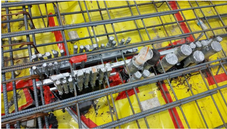
Slab with grade beams in lower left and upper right. #6 at 12" in direction of span. Utility boxes are mounted on big 4000 psi blocks. Rebar on 4000 psi bricks.
