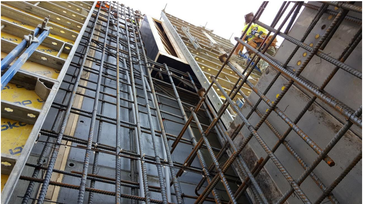
Inspecting Wall Corners before forms are closed
