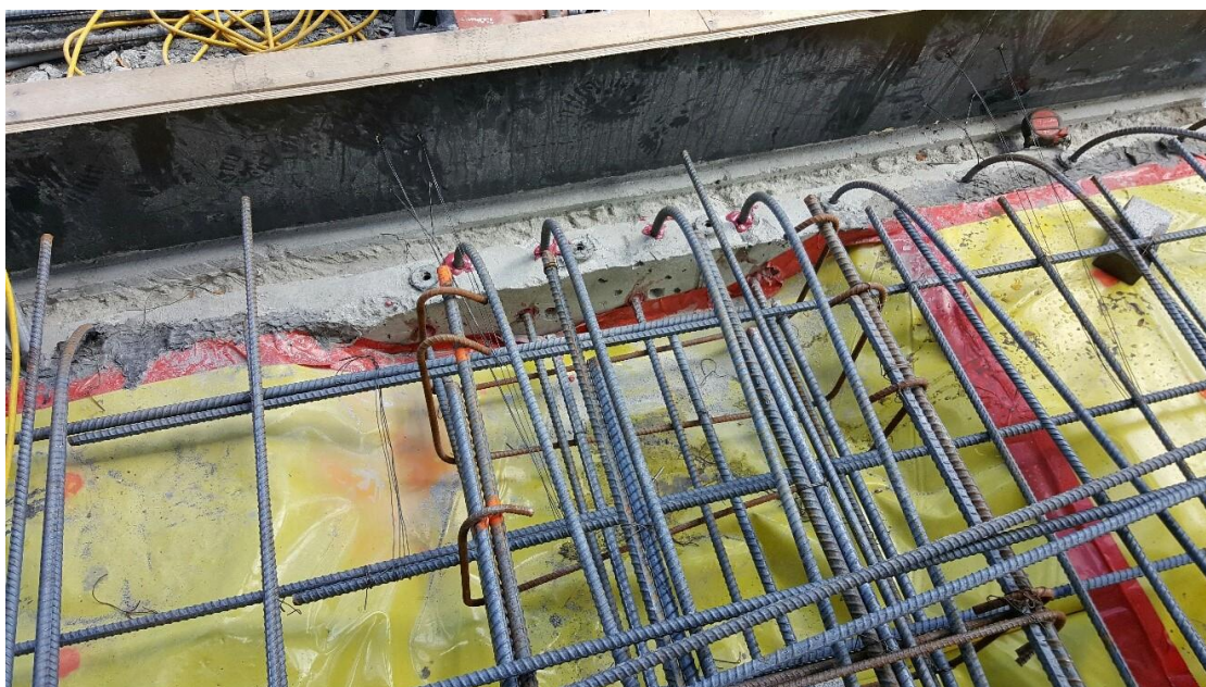
Dowels as form savers & as drilled and epoxied at slab on grade and grade beam. Additional top and bottom bars were added above the bent dowels.
