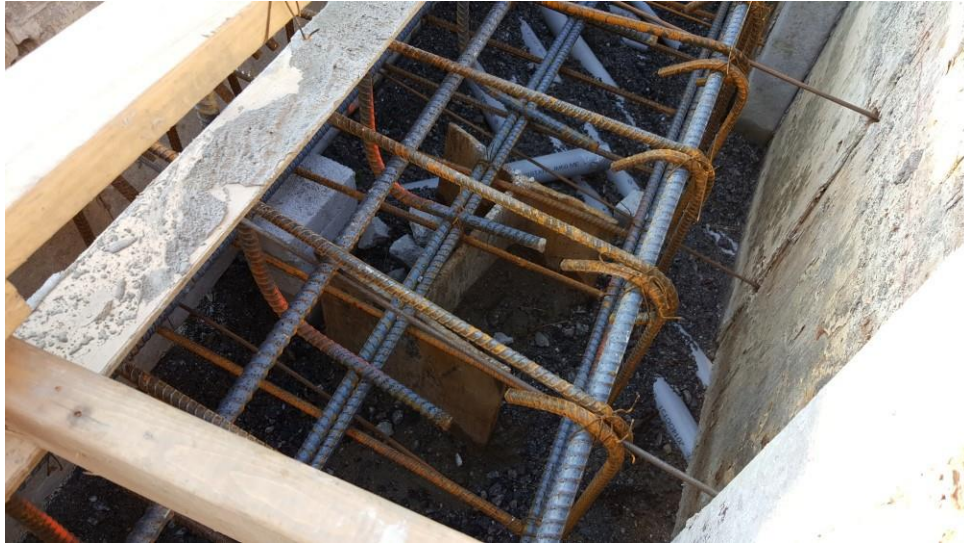
Grade Beam Rebar with 135 degree bent Stirrups over a Pile
