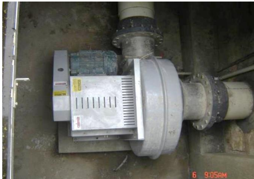
Figure 18: Looking down on a blower that draws odorous air from the right and discharges the air at a higher pressure through the pipe at the top.
