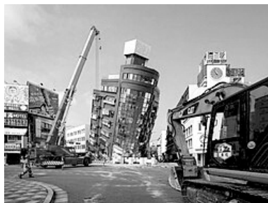
Semi-collapsed building - 2024 Hualien earthquake, China.
