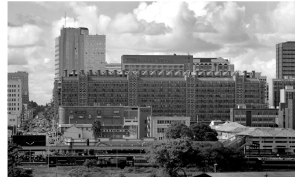
Figure 4.33. – The Eastgate Centre Shopping Centre & Office Building; The building is ventilated and cooled entirely by natural means. © David Brazier – Wikipedia
