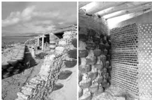
Figure 4.16. - Earthships (global) made of tire walls © nbcnews
