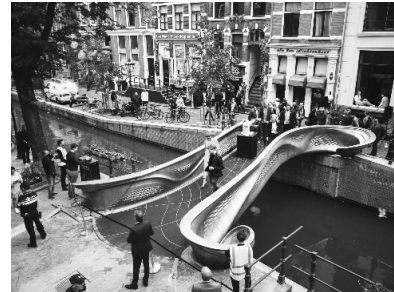
Figure 4.17. - MX3D 3D-printed steel bridge, Amsterdam (2021) © friedmanbenda.com
