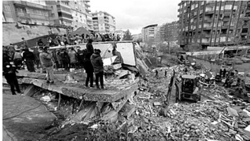
2023 Turkey Earthquake Damage Diyarbakir
