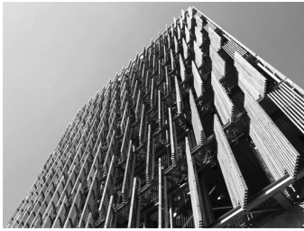
Figure 4.22. - CH2 - Council House 2, Melbourne © inhabitat.com
