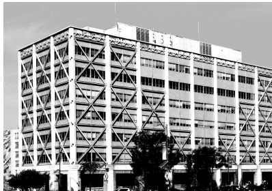
UC Berkeley University Hall retrofit with seismic façade;
