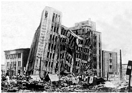
Fukui Earthquake 1948 - damaged building.
