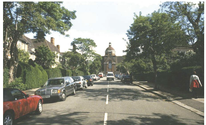
Figure 1.1. Hampstead Garden Suburb, London, begun 1907. Master plan by Barry Parker and Sir Raymond Unwin. The Free Church (at end of axis) by Sir Edwin Lutyens (1908-10). Note how the urban designers place a significant civic building to close the axial view and intensify the “sense of place.” Photo: David Walters
