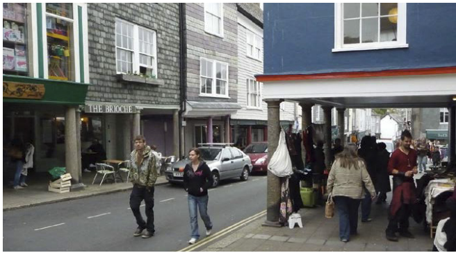
Figure 3.7. The “Butterwalk,” medieval shopping colonnade along the High Street in Totnes, U.K. Originally designed to cover market stalls, this use continues today for retail and restaurant activity, providing very rich and active edges to the public space. Photo. David Walters.
