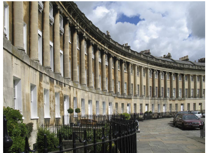
Figure 3.3. The Royal Crescent, Bath, UK. 1767-74. John Wood the Younger, architect. The front façades of thirty town homes are reconceptualized as a unified composition at the scale of a royal palace – a brilliant real estate development strategy married with excellent design. Photo. David Walters.
