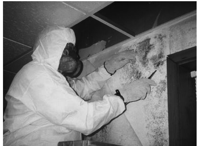
Use of additional personal protection equipment
