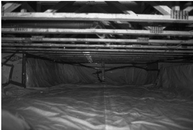
Properly protected crawl space
