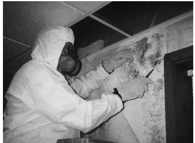
Use of additional personal protection equipment
