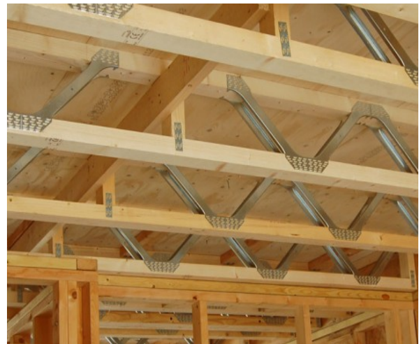
Floor Truss Framing
