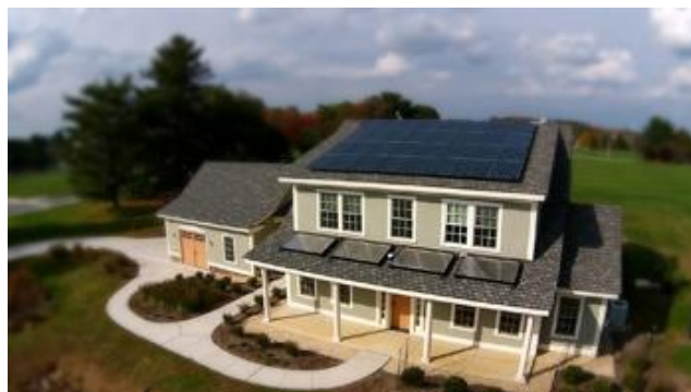
Figure 3 NIST Net-Zero Energy Residential Test Facility
