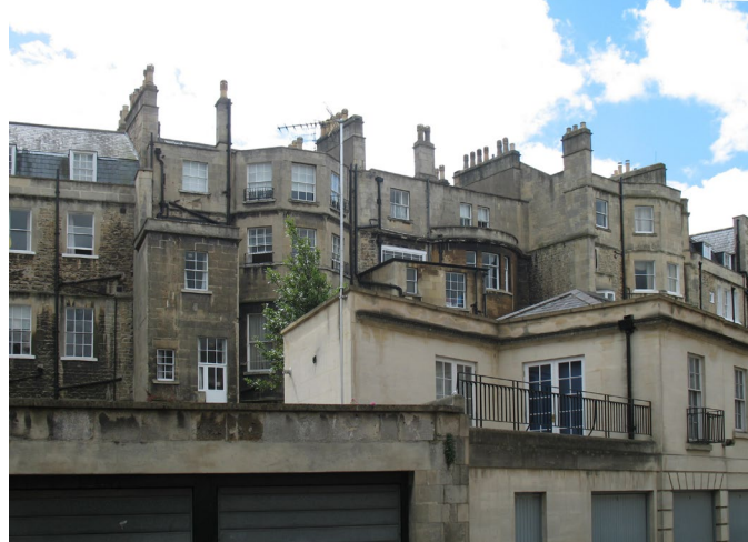
Fig. 15. Rear Façade, Royal Crescent, Bath, UK. Generations of alterations and additions have created an informal arrangement that is the antithesis of the front, but which perfectly suits the rear service street. Photo by David Walters
