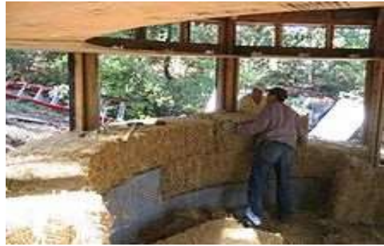
Building with Straw Bales
