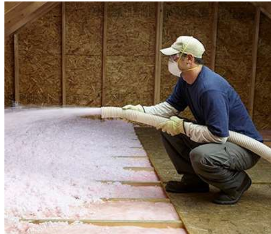
Blowing In Insulation
