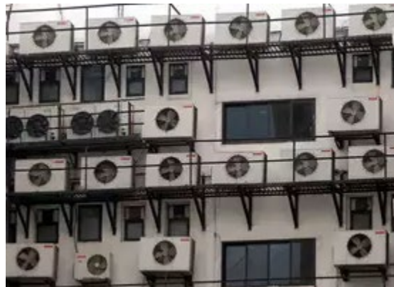
AC units overtake the building facade
