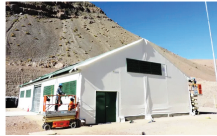
(Image courtesy of Legacy Building Solutions.) Explosives storage for a mining facility in the Atacama Mountains, Chile.
