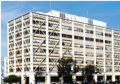
UC Berkeley University Hall retrofit with seismic façade; Source: Interactive Resources
