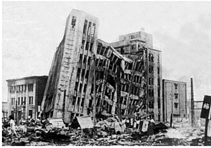
Fukui Earthquake 1948 - damaged building.
