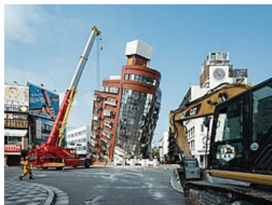
Semi-collapsed building - 2024 Hualien earthquake, China.
