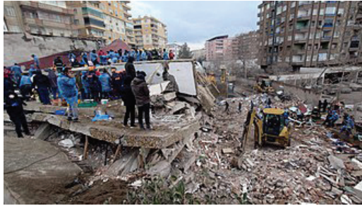
2023 Turkey Earthquake Damage Diyarbakir
