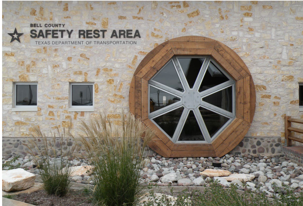
Bell County Rest Area (2008), Jarrell, Texas; TxDOT Roadside Facilities Design Group; Photo: courtesy of the author; © Muhammad A Siddiqui 2008.
