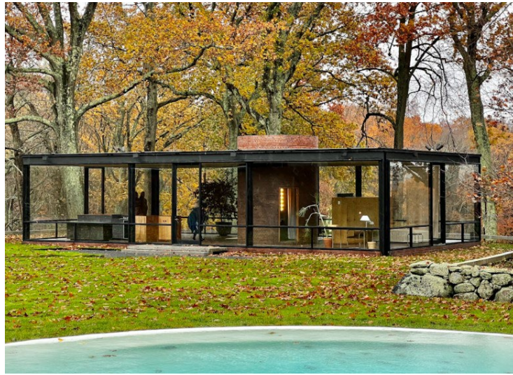
Edith Farnsworth House (1946-51); Mies Van Der Rohe; Photo: Wikimedia Commons: Farnsworth House Interior.jpg
