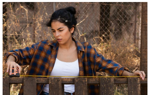
Figure.77. Tradesperson repairing a residential fence. Los Muertos Crew/Pexels.com
