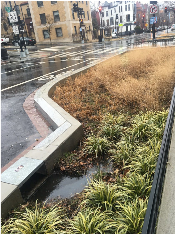
" Street drainage into bioswale " by Eric Fischer is licensed under CC BY 2.0 .
