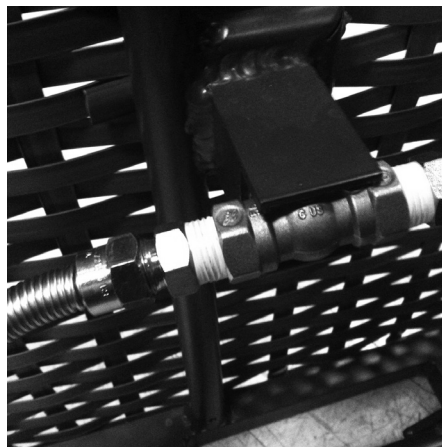
Fig. 14 Attach end of 1/2" flex connector to manual gas valve.
