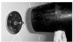
14. Verify the length of the nut from the **WingIt** faceplate is correct (step 8) – Then hit the **WingIt** firmly with a rubber hammer.
