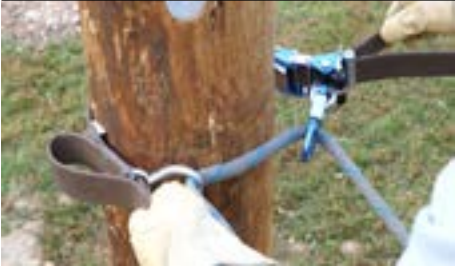
Figure 7A: Moving Strap Adjuster Towards Pole
