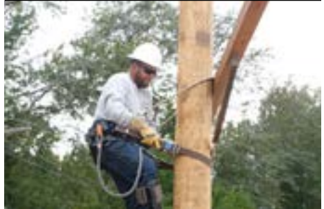
Figure 23: WPFRD Installation below Obstruction
