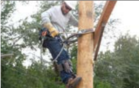
Figure 22: Secondary Rope Installation
