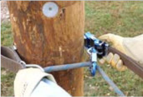
Figure 8: Moving Strap Adjuster Away from Pole
