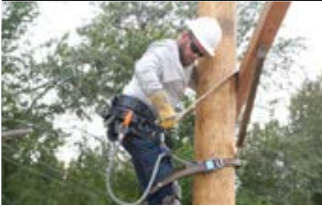
Figure 20: Secondary Rope Device Installation
