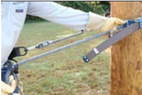
Figure 14: Moving Rope Adjuster Towards Pole
