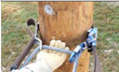
Figure 13: Acceptable Inner Rope Orientation
