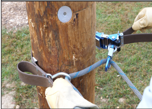
Figure 7A: Moving Strap Adjuster Towards Pole
